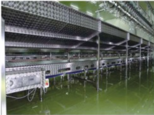
Production boxes conveyor at weighing line
