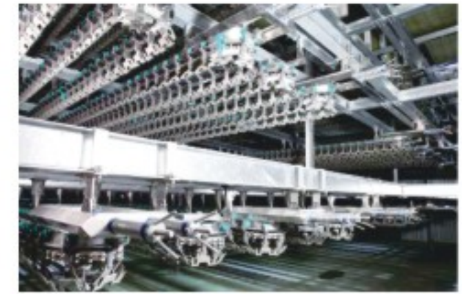
Air chilling at side
