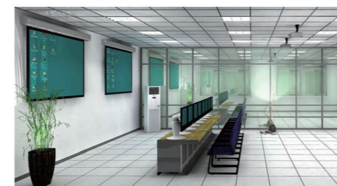
Centralized Control Onsite
